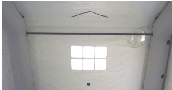
Figure 2.7 - Spacer rod (PURLIN) installed.
