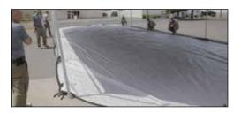
➤ Working around the perimeter of the shelter, gently lift the frame and pull the floor panel under it. Center the shelter legs on the black reinforcement patches. Pull out on the corners to flatten the floor.
